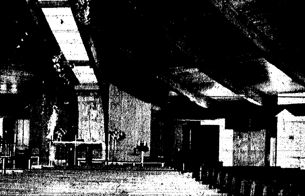
THE CEILING of St. Mary's new church is supported by massive laminated wood beams. The building is in the shape of a diamond, with skylights forming a cross in the roof. The new church seats 700 and does not include extra facilities for education or other activities. The choir and organ locations may be seen to the left and right of the sanctuary. Contemporary stained glass windows are placed along the sides of the church.
